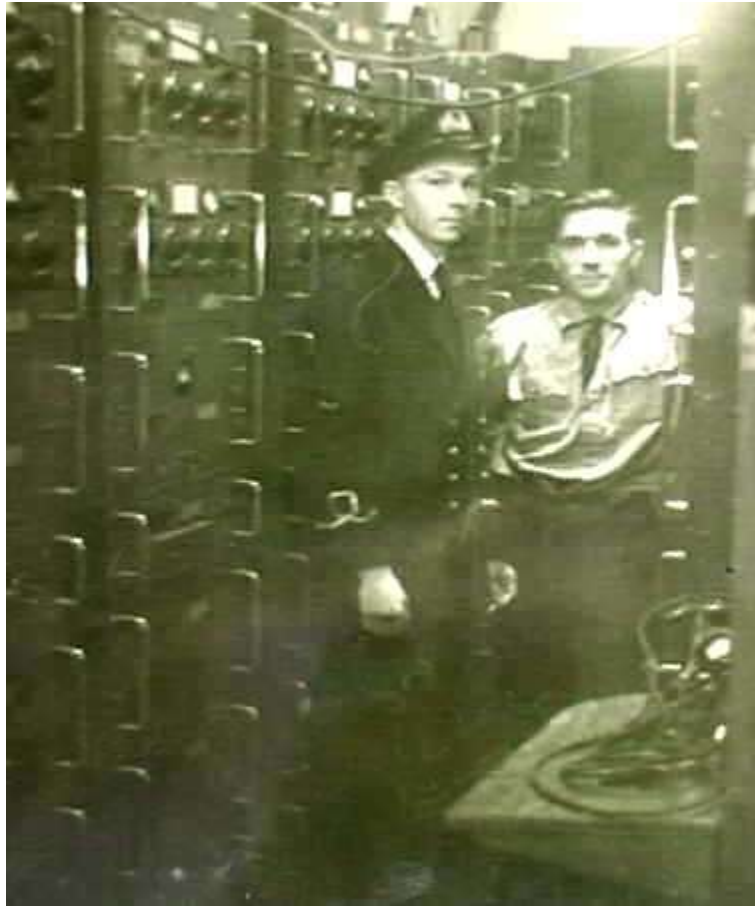
FDT transmitter room
